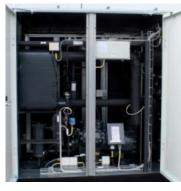
Cooling compressor with automatic capacity regulation and heat exchanger. Type of refrigerant, 14-16 kg R407C depending on the size of the cooler.
