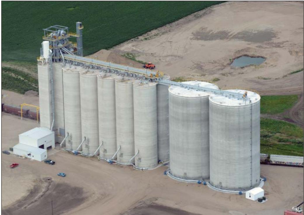
*The Hamberg, LLC 2013 rail terminal in Hamberg, ND is a joint venture between CHS and Fessenden Coop Association. One-million-bushel slipform concrete annex at right was completed at the beginning of 2015. Aerial photo courtesy of Vigen Construction Inc.*
