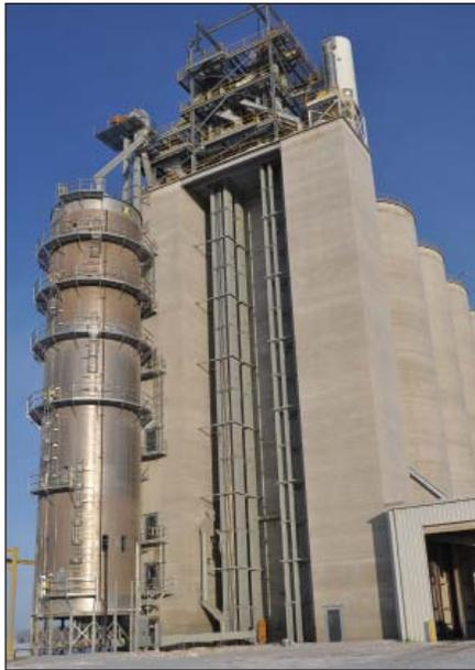
*The Hamberg terminal operates five bucket elevators seen in alcove and a 7,000-bph Zimmerman tower dryer at left.*
