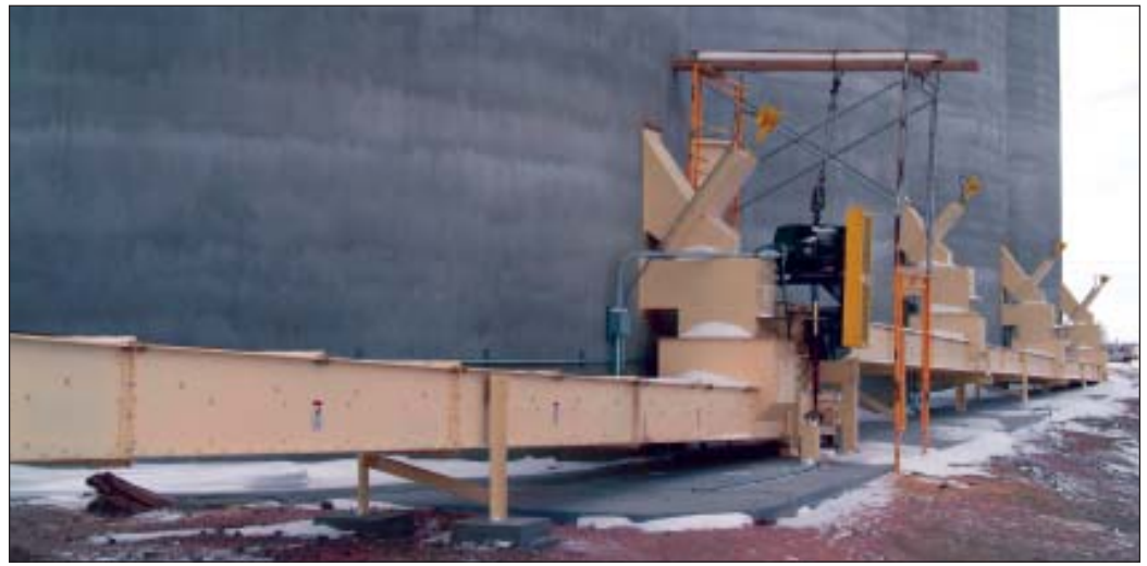
A series of sidedraw outlets allow grain to empty onto a series of Essmueller drag conveyors. When grain drops below the level of the sidedraws, it drops through air-assisted Kanalsystem floors.
