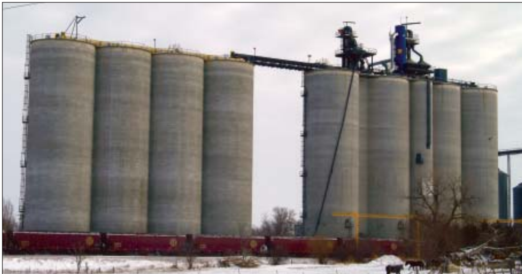
Cargill AgHorizons' rail-loading terminal at Emery, SD, with a new four-tank slipform concrete annex at left. Photos by Ed Zdrojewski.
