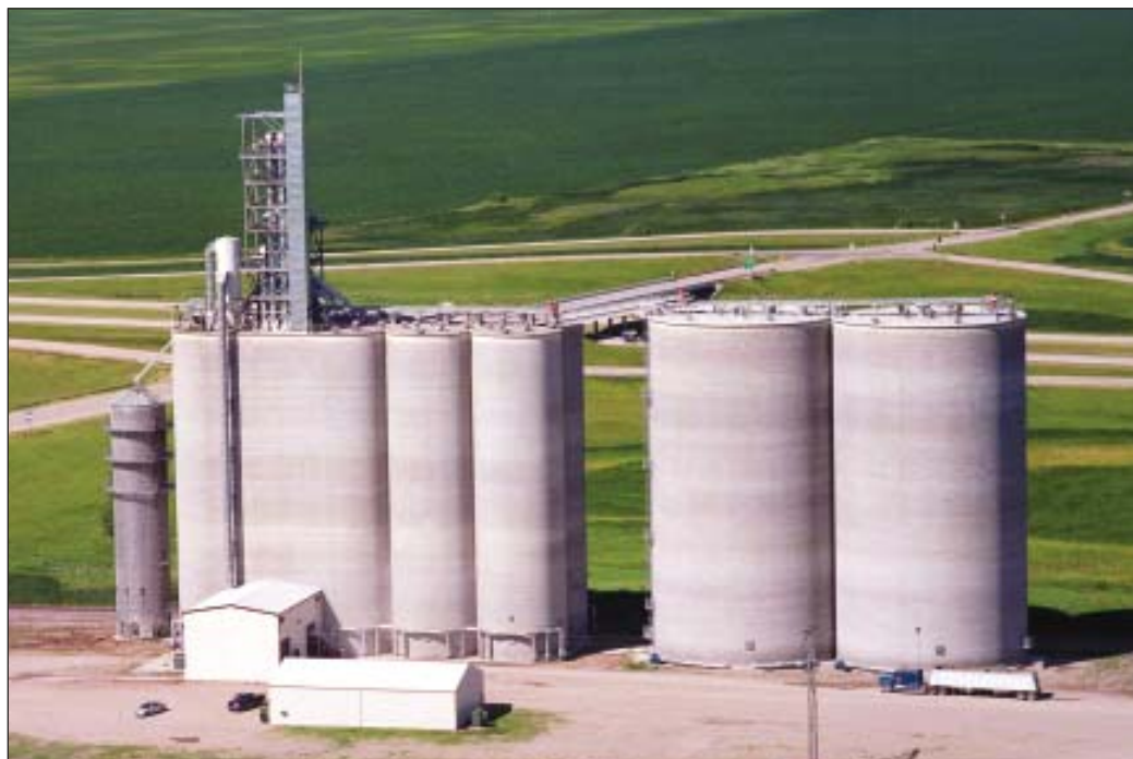
Alton Grain Terminal LLC's shuttle-loading grain terminal south of Hillsboro, ND, with two new 500,000-bushel slipform concrete tanks at right. Aerial photo courtesy of Vigen Construction Inc.
