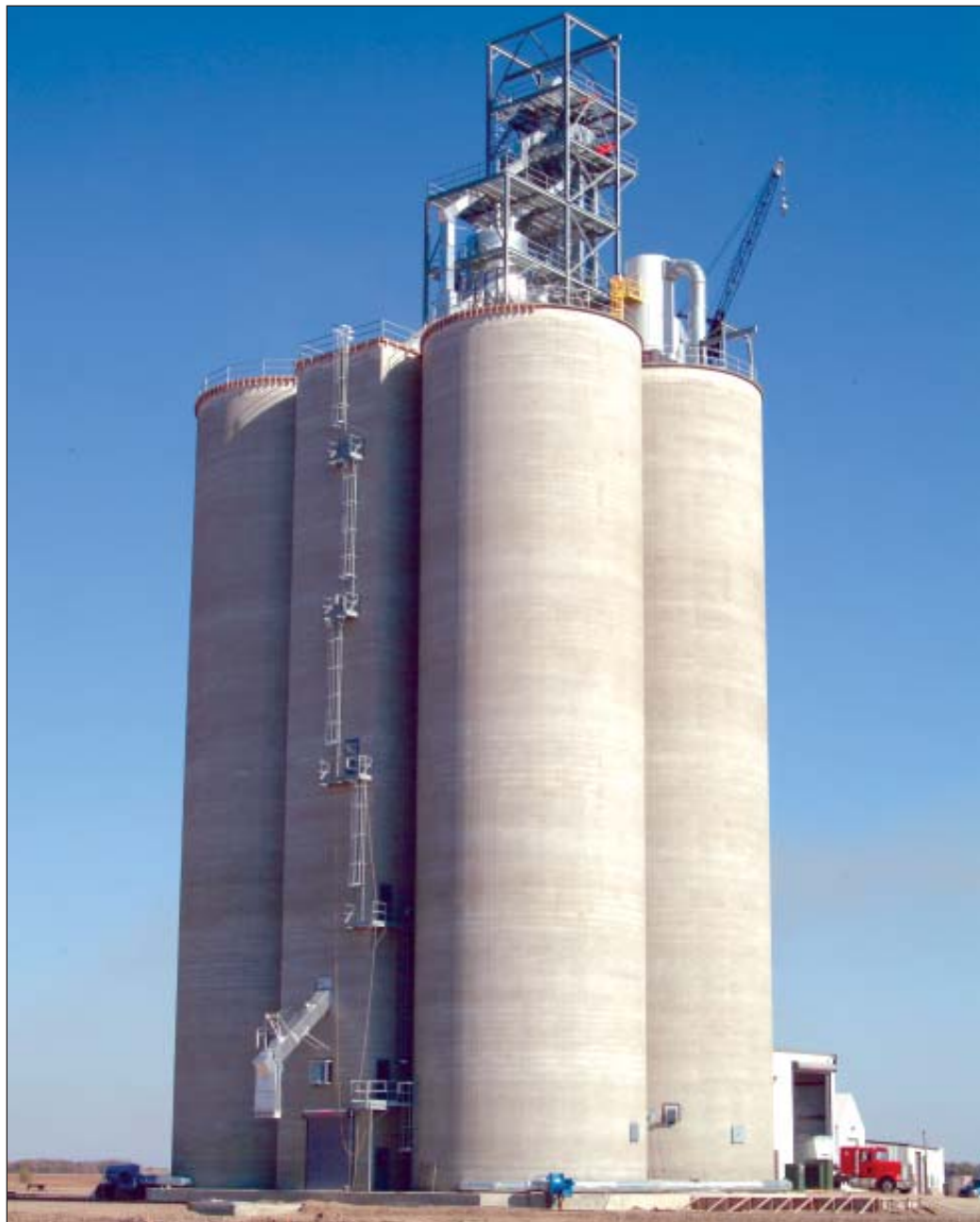
BTR Farmers Cooperative's new 680,000-bushel rail-loading terminal near Leeds, ND, can load 110-car shuttle trains in 10 hours or less. Photos by Bruce Selyem.
