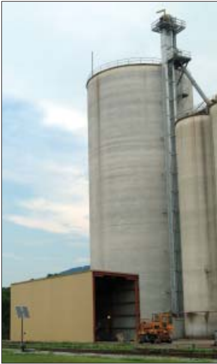
From left, new enclosed rail receiving pit, 300,000-bushel slipform concrete tank, and 20,000-bph Essmueller leg were all part of the upgrade.
