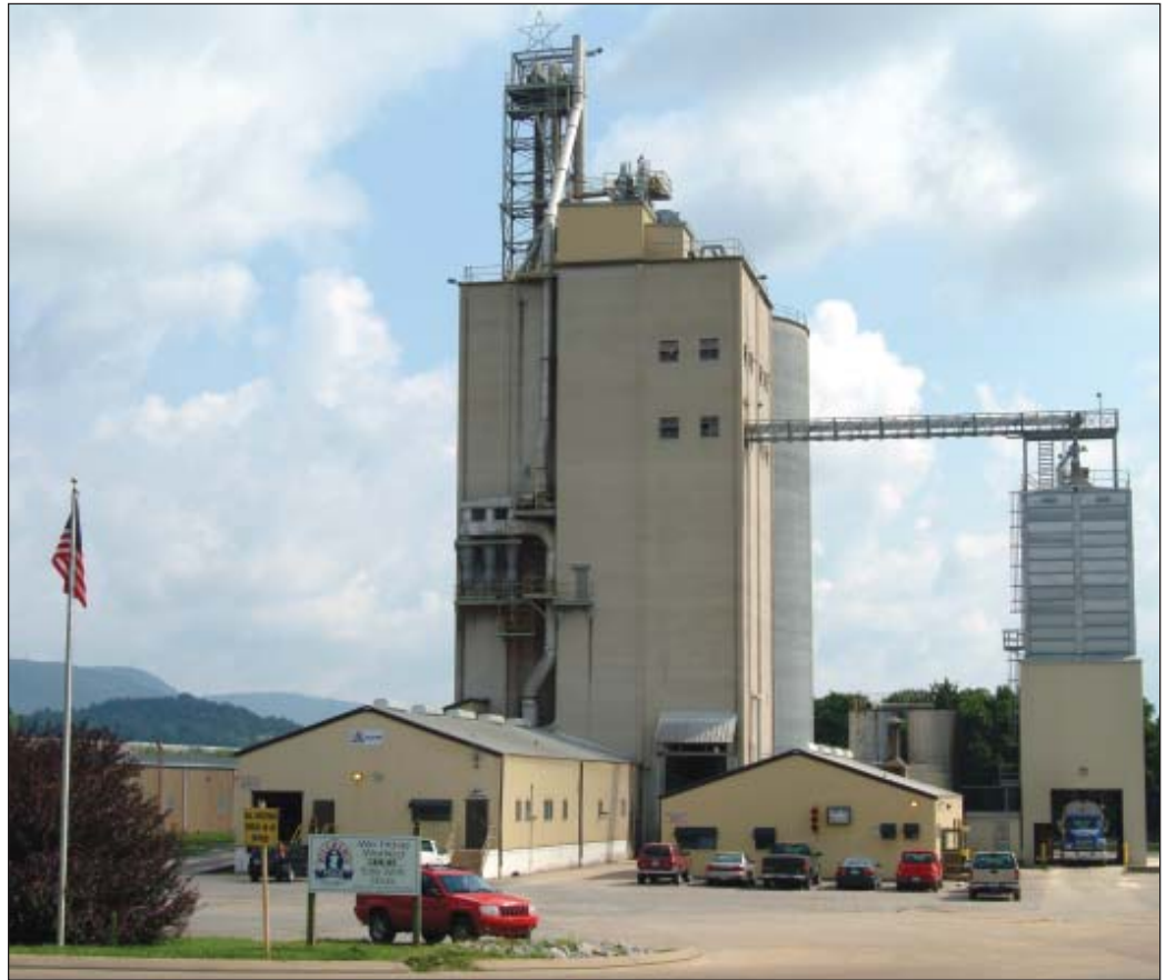
Pilgrim's Pride Inc.'s 120-tph feed mill at Chattanooga, TN, acquired in 2003 after the previous owner, ConAgra Foods, upgraded it from 70 tph. Photos by Ed Zdrojewski.
